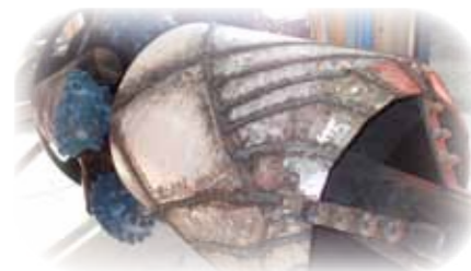
▲ 1050mm diameter tunnel requiring three reamer passes
