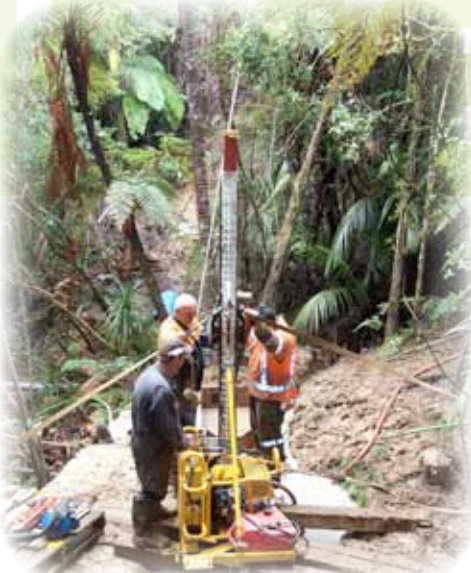
▲ Heli rig used for grout injection and additional ground investigation
