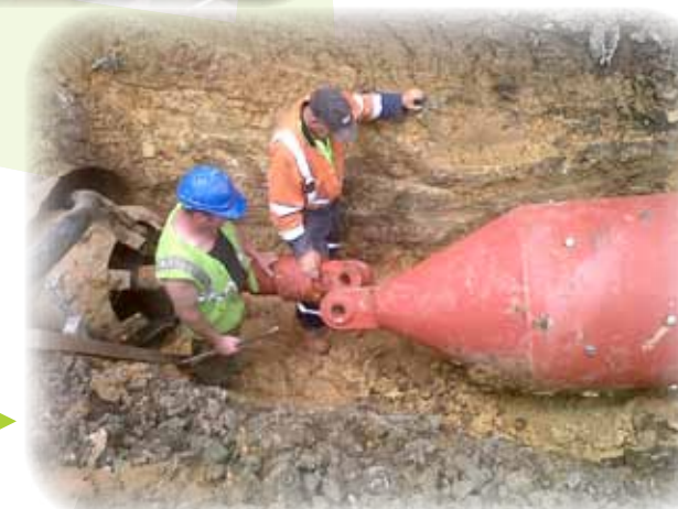
▶ Connecting the towing head to the swivel
