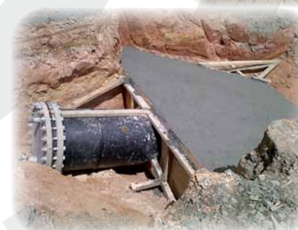
◀ Anchor block construction
