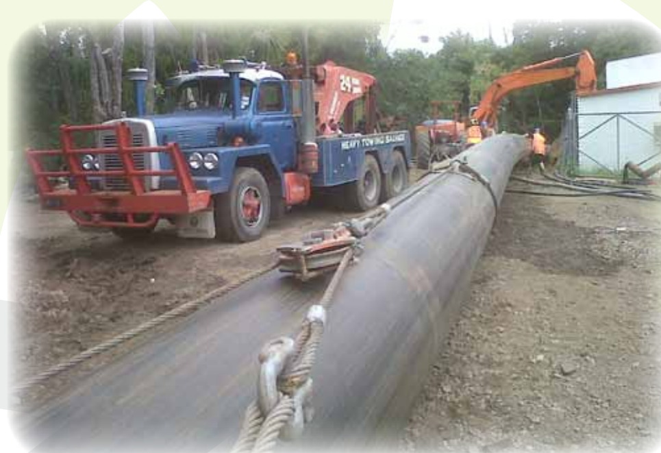
▲ Maneuvering 200 ton of pipe required plenty of grunt
