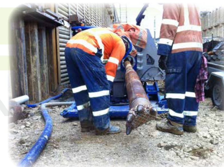
▲ Non-magnetic tooling fitted with ParaTrack II and DCI Eclipse location sensors.
