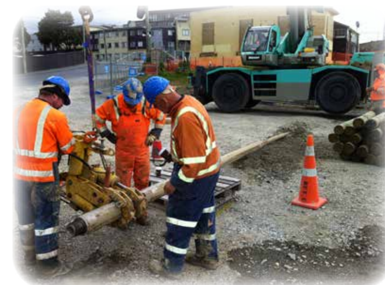
▲ Removing the non mag drilling head with the scorpion pipe wrench.
