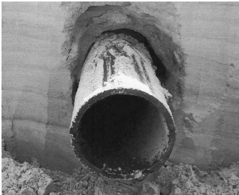
Fig. 9. 200 mm (8 in.) sand excavation at 1 day
