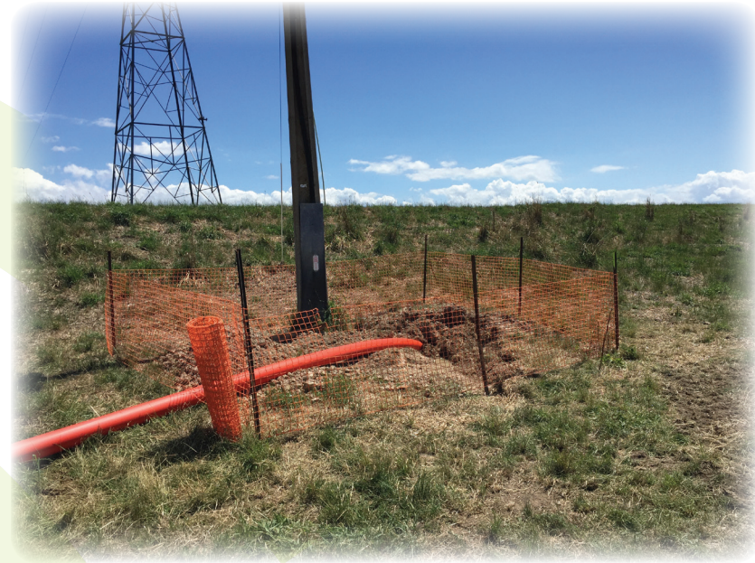
▲ Pipe string entering the ground on the East Side of the river
