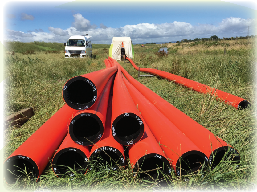
▲ 160mm diameter PE pipe in 17m lengths welded into a 500m long pipe string.
