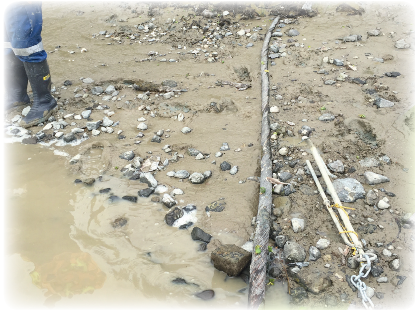
▲ Existing power cable dangerously exposed on the west bank of the Waihou River.
