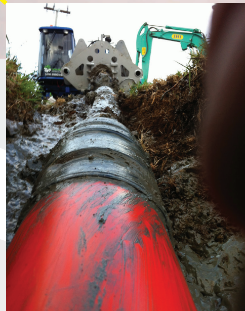
▲ Pipe exiting at drill after crossing under the river.
